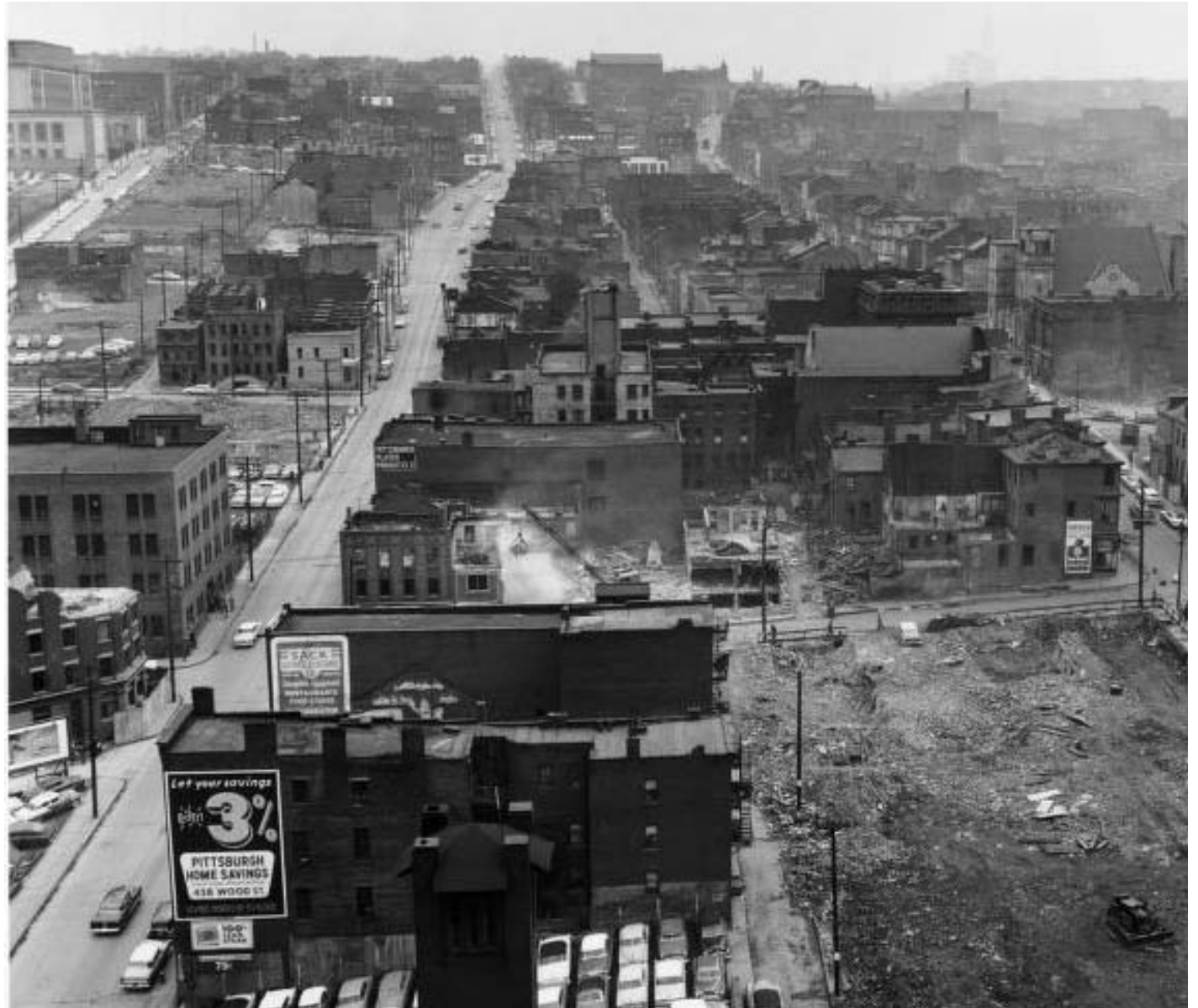
Beginning of demolition of the Lower Hill, ca. 1955. Source: Allegheny Conference on Community Development Photographs, 1892-1981, MSP 285, Library and Archives Division, Senator John Heinz History Center
