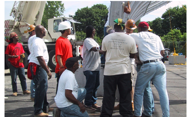
Construction/Renovation/Historic Preservation: Construction could play a pivotal role in workforce development in the Hill District.
