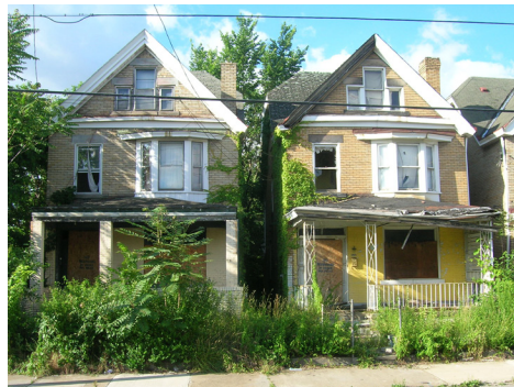
Vacant Houses on Tioga Street
