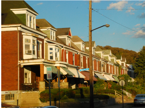
Renovation of Existing Housing
