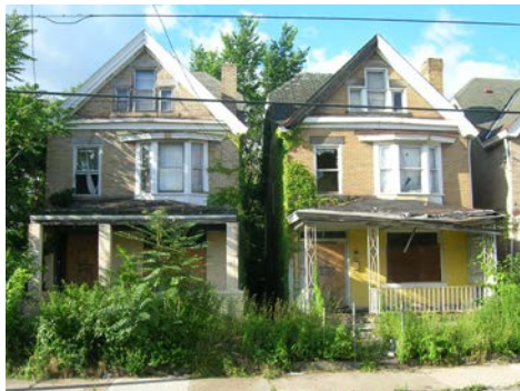
Vacant Houses on Tioga Street
