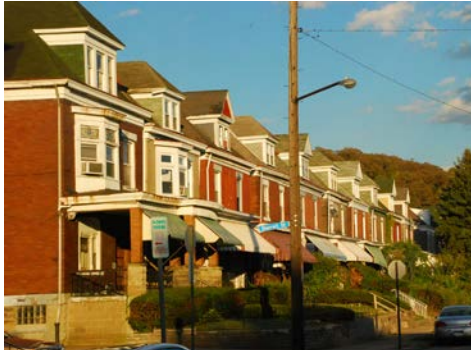
Renovation of Existing Housing
