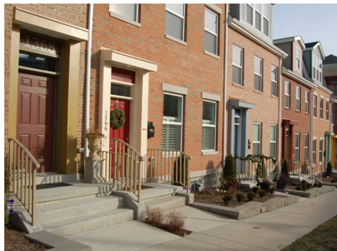
New Affordable Housing: Federal Hill on Pittsburgh's Northside
