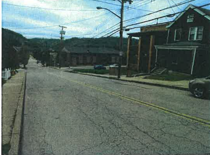
HAZELWOOD AVENUE LOOKING NORTH SUBJECT AT LEFT
