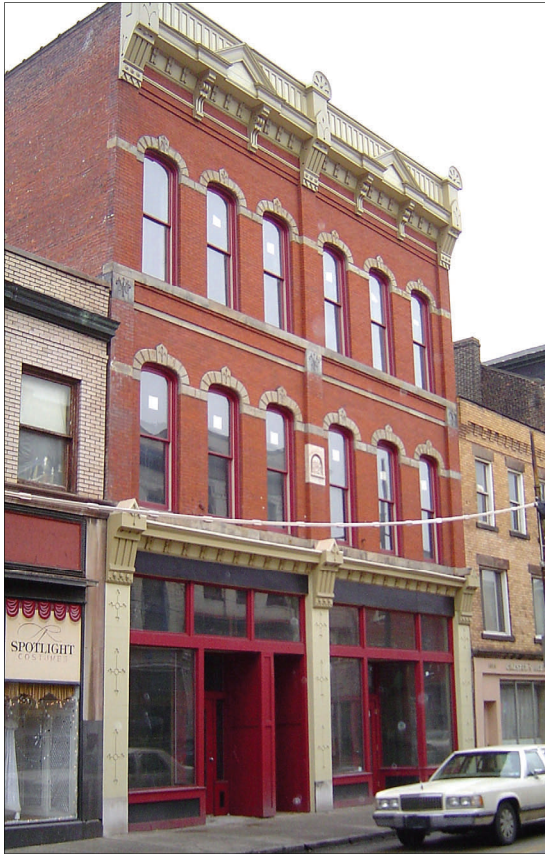
Figure 24. Brick façade cleaned and repointed
