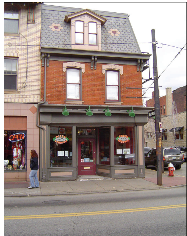
Figure 27. Mansard roof restored with slate
