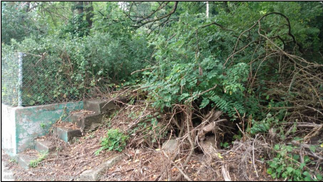
Former foundation found on Subject Property
