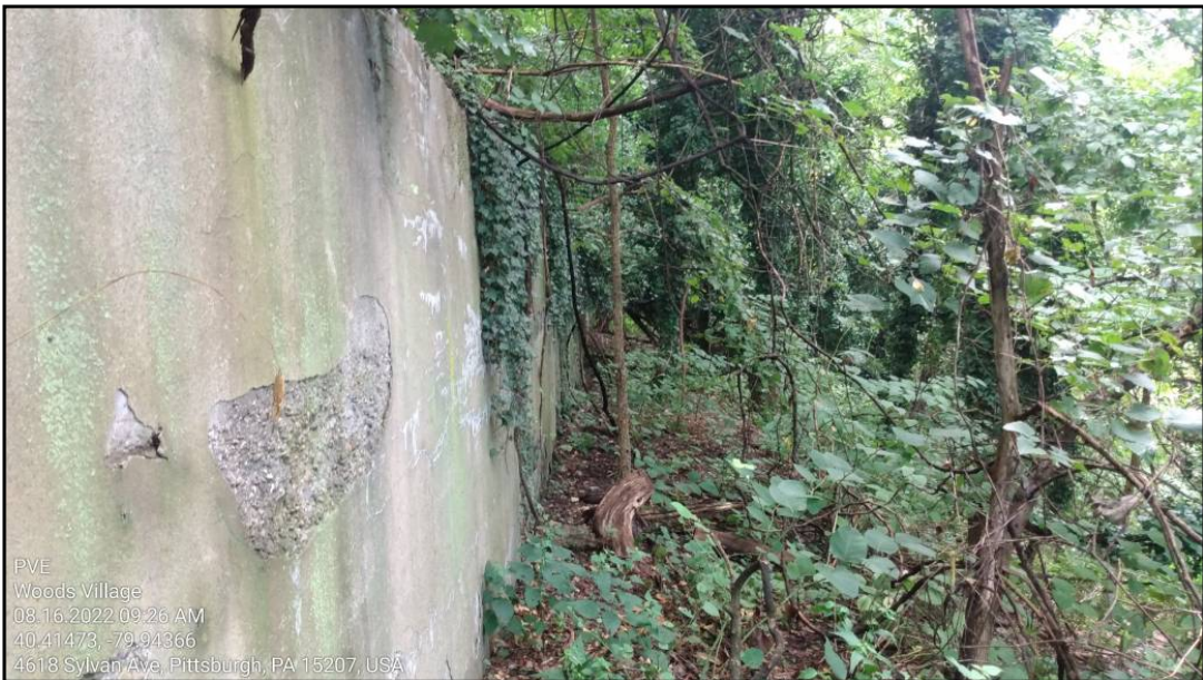
Foundation wall of former rowhouses
