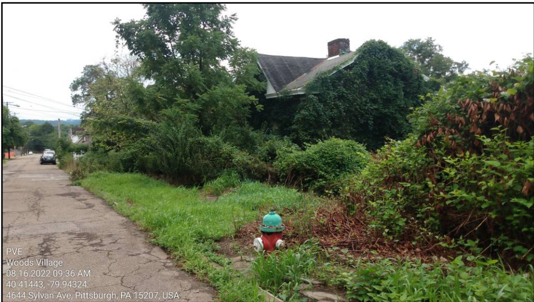
Abandoned structure at 4656 Sylvan
