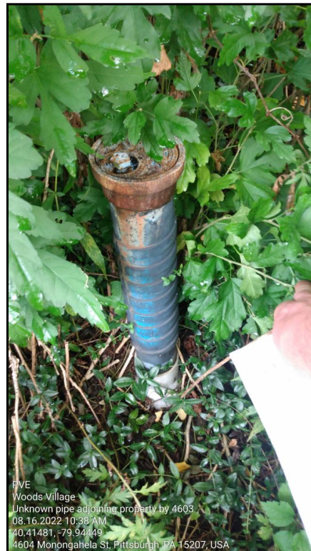
Unknown water pipe on adjoining property on Monongahela St.
