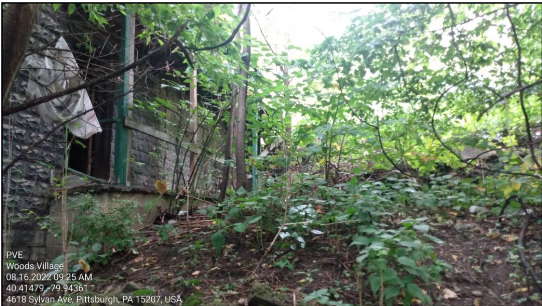
Typical structure side
