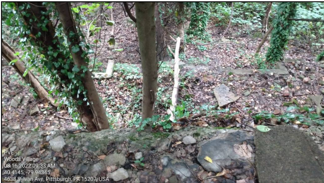
View of wall from above
