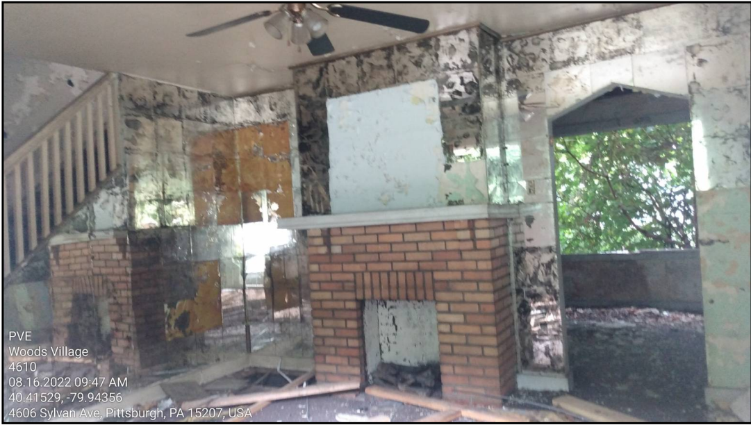
Abandoned structure interior example
