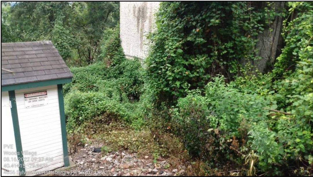
Stressed vegetation surrounding natural gas shed
