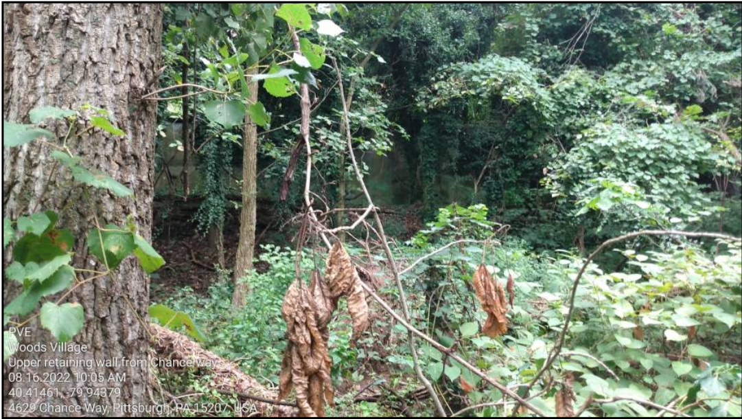
Foundation wall viewed from Chance Way
