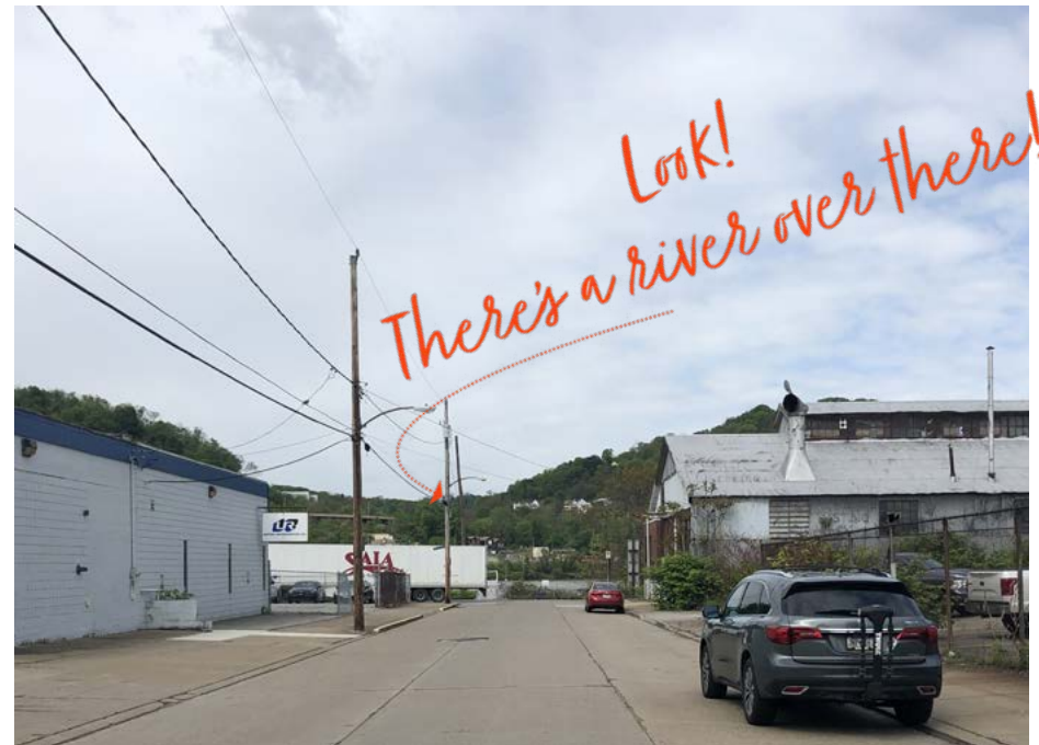
North Franklin Street today
