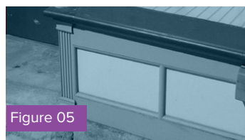
Figure 05. Paneled wood bulkhead panels below display windows
