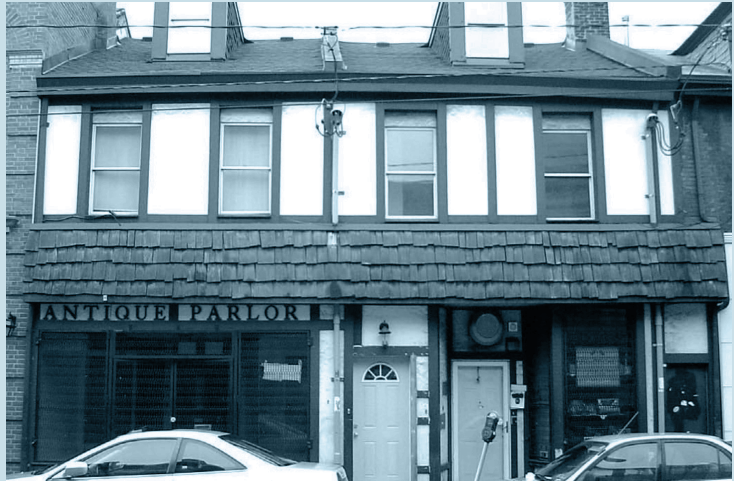
Figure 03. Inappropriate remodeling: inauthentic Tudor details added to a Greek Revival building
