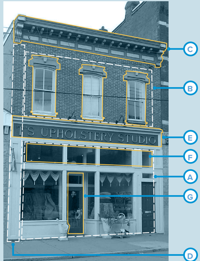
Figure 01. A typical traditional commercial building (overlay: evolveEA)
